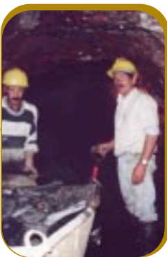
Refurbishment work at Banjas Mine
