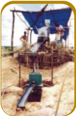
Small mobile plant
